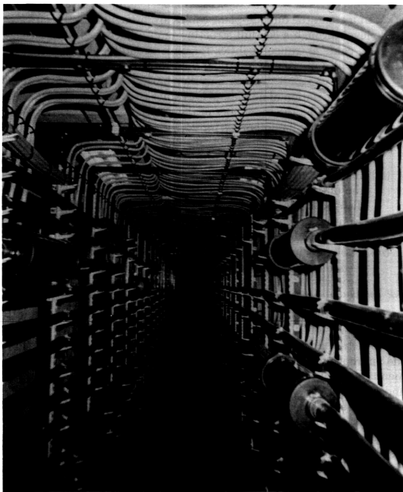
Fig. 12—A subgrade cable entrance facility with provision for cable penetration through basement walls, ceiling, and the outer wall to upper floors.
