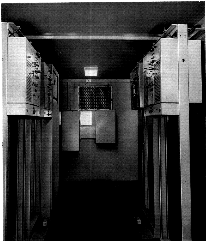
Fig. 64 — Interior view of an equipment shelter at a repeater station equipped for a diversity message system (ultimate capacity is 3 diversity systems).
