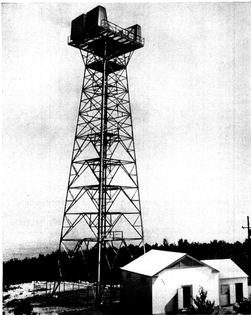
FIG. 10—Microwave radio relay tower at Cotoctin Mountain, Maryland, on a New York-Washington radio route. There are 300 message circuits in service with more planned.
