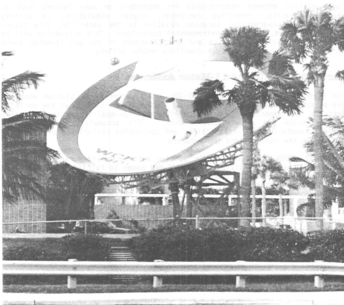
Figure 1. Scientific-Atlanta 10-Meter-Diameter Earth Station for Video Transmitting and Receiving
