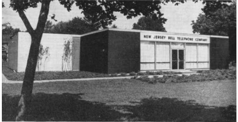
The Bell System's first commercial electronic central office is housed in this building at Succasunna. It began serving 4300 New Jersey Bell Telephone Co. customers on Sunday, May 30, 1965.
