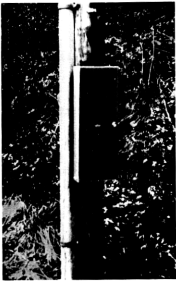
Fig. 18— SLC ™ -40 pole-mounted repeater enclosure.
