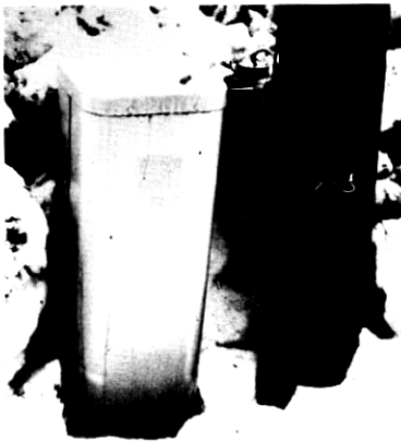
Fig. 19— SLC ™ -40 pedestal-mounted repeater enclosure.
