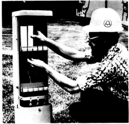
Fig. 19— SLC ™ -40 pedestal-mounted repeater enclosure.
