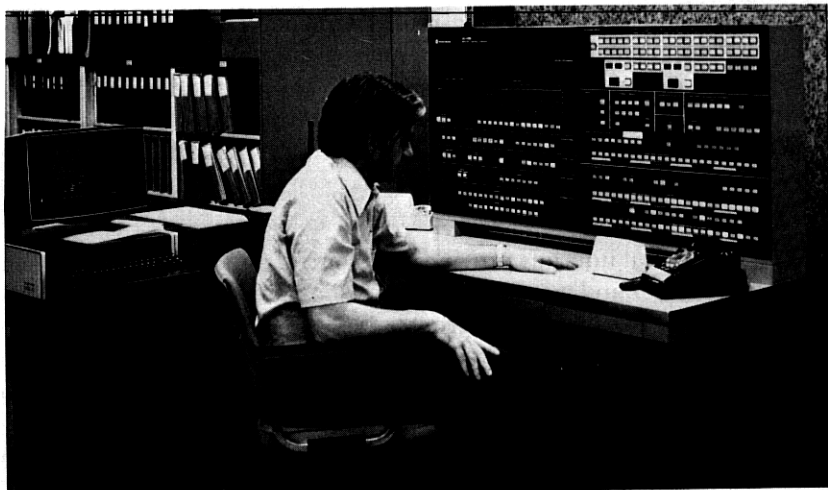
Fig. 13—Master control console.
