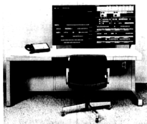
NO. 4 ESS MASTER CONTROL CONSOLE
