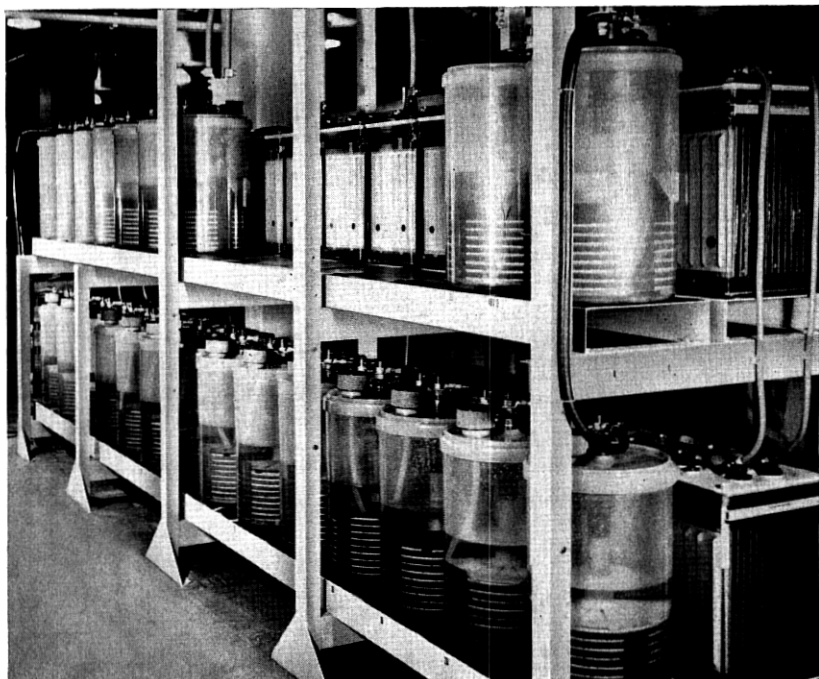
Fig. 8—Early trial installation of new cells.
