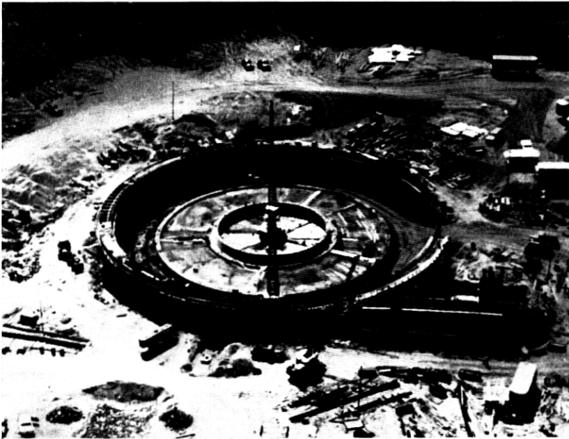
Fig. 8 — Completed antenna foundation and partially constructed foundation for attachment of radome.
