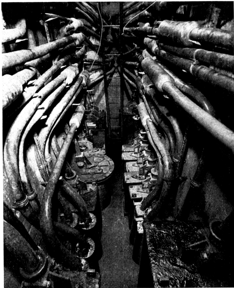
Fig. 28B—Other end of vault in Fig. 28A.
