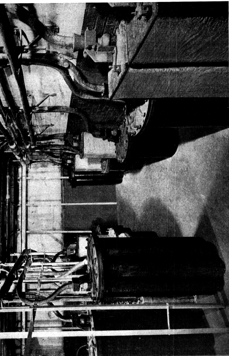
Fig. 26—Office vault installation of exchange area trunk cable loading. This vault is in the basement of a Manhattan office, close to the East River. The coils are used for loading trunks between Brooklyn and Manhattan offices routed through cables which cross the river in a rapid transit tunnel where space restrictions prevent the installation of loading coil cases. At time of photograph, a total of 36 cases containing a total of 11,404 coils were installed in this vault. The 36 cases comprise 20 cast iron, 9 rectangular welded steel, and 7 tubular thin steel designs. The view shows 17 cases; the other cases are hidden in background or are out of camera range. One case contains 456 coils; in the others the complement ranges from 303 to 306 coils. The individual coil codes are 601, 602, 603, 612, 613, 614 and 632. About 13% have iron dust cores, 63%
