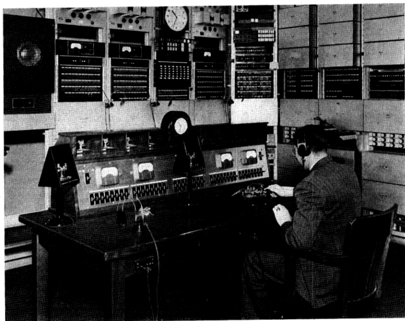
Fig. 5—Monitoring position at Washington, D. C.
