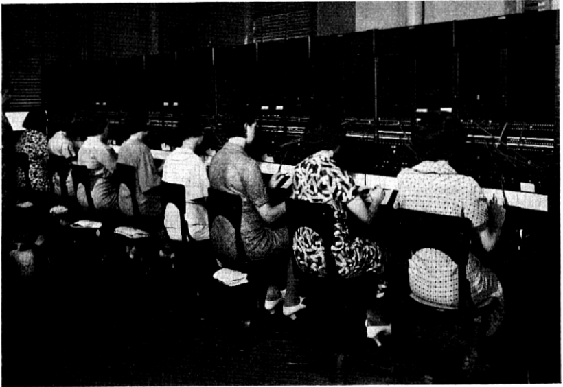
Fig. 6—No. 3A Teletypewriter Switchboard at Pittsburgh, Pa.
