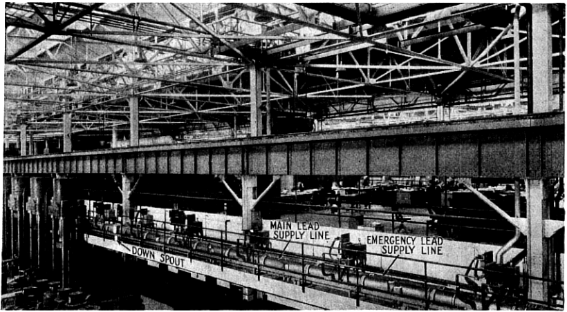
Fig. 28—Main lead supply lines.
