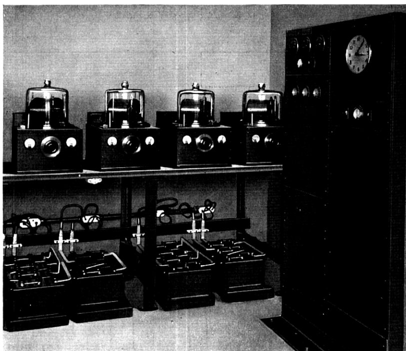
Fig. 17—Four 100,000-cycle oscillators with auxiliary equipment.
