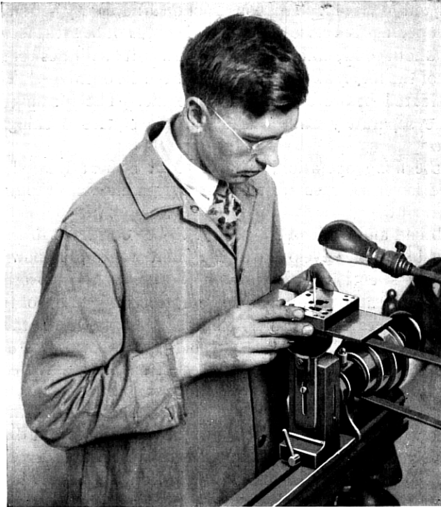
Fig. 18—Filing out die openings with filing attachment on bench lathe.
