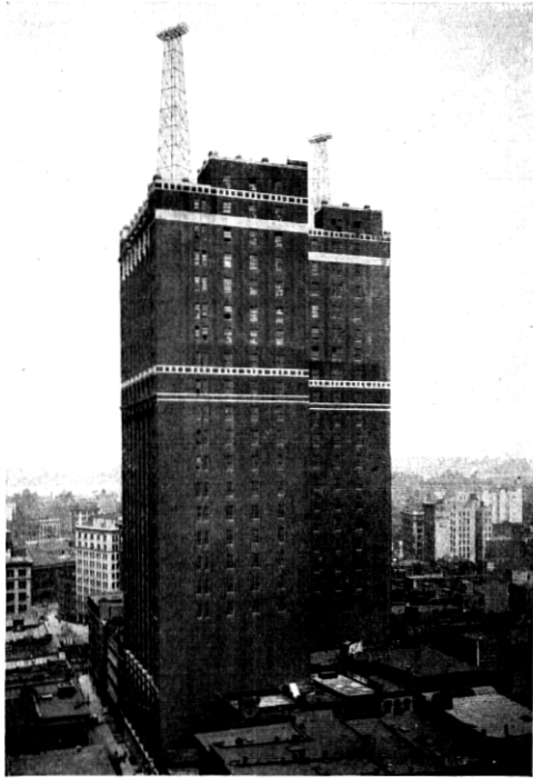
Fig. 17—Long distance telephone building, New York City
