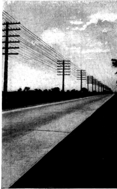
Fig. 2—Open wire toll line
