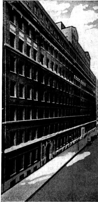
Fig. 16—West 36th Street building, New York City
