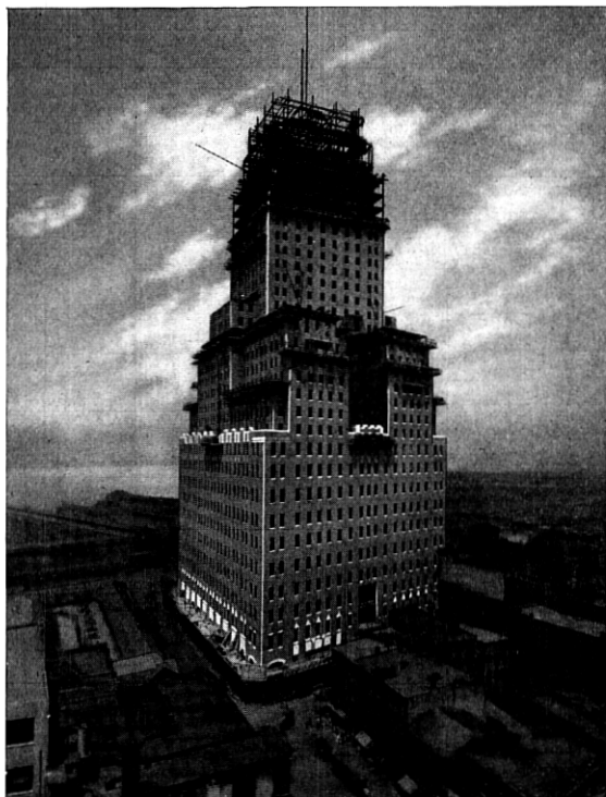
Fig. 18—Barclay-Vesey telephone building under construction, New York City
