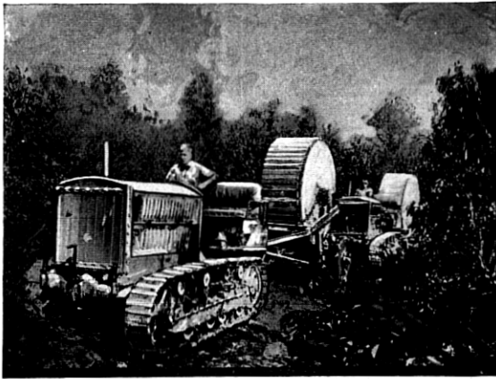
Fig. 3—Transporting cable reels through Allegheny Mountains
