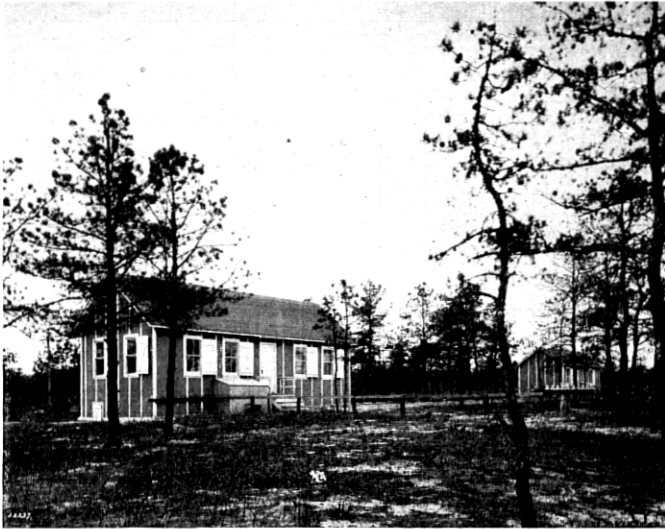
Fig. 2—Exterior of Riverhead Radio Receiving Station
