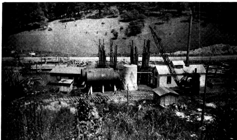
Fig. 22—View of Treating Equipment at Sylva Plant
