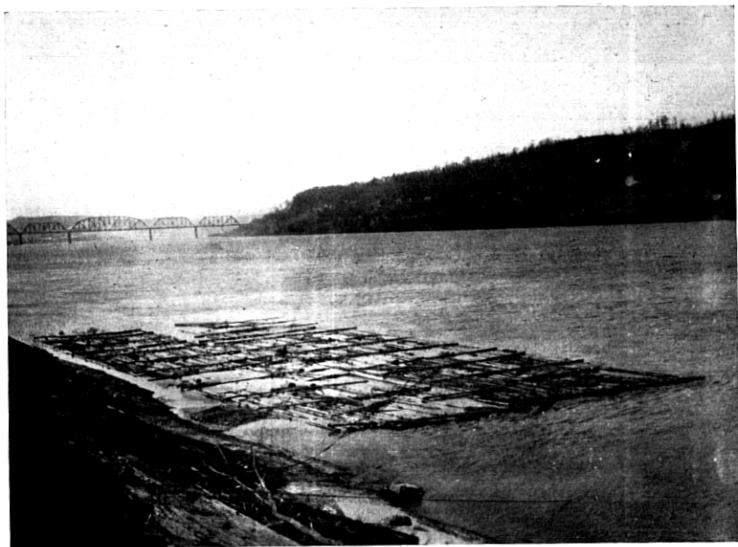
Fig. 10—Four Rafts of Poles at Ceredo Plant
