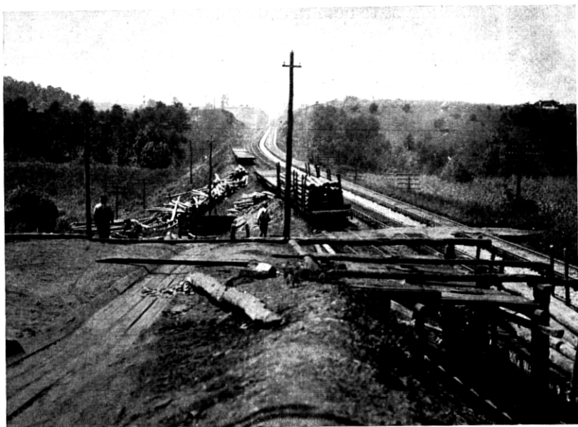
Fig. 9—Unloading Poles at the Shipman Yard
