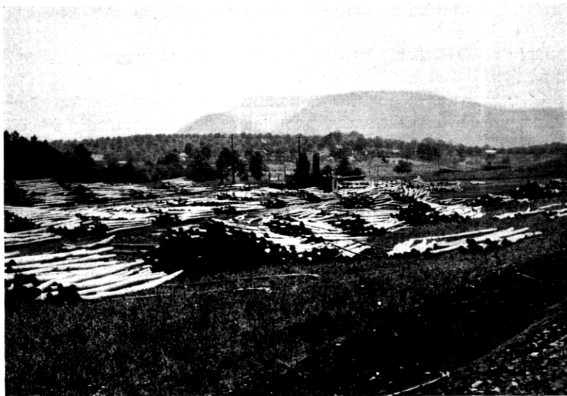
Fig. 31—General View of Natural Bridge Plant in Operation
