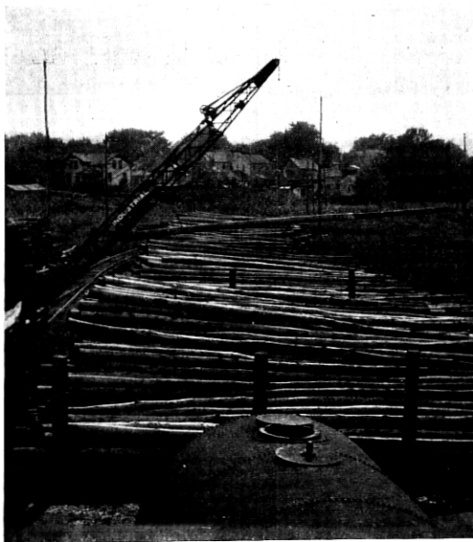
Fig. 18—Handling Pole with End Butted Against Boom of Locomotive Crane
