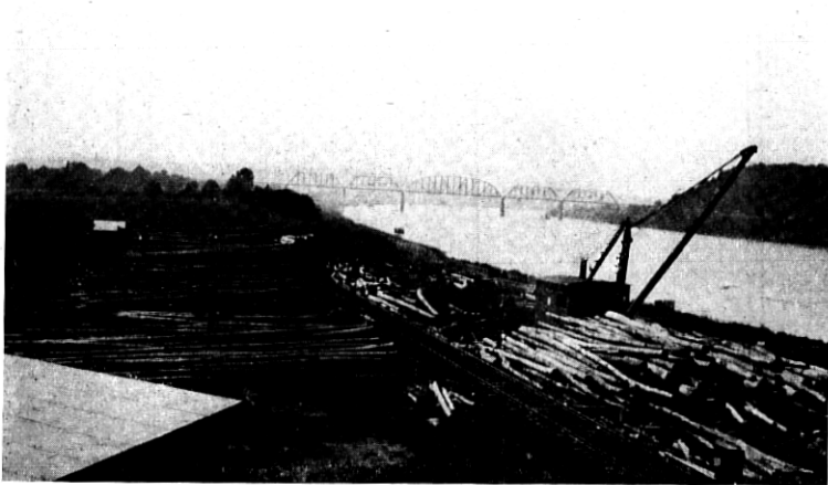
Fig. 12—Derrick for Handling Poles from River Rafts to Piles or Pole Cars in the Yard
