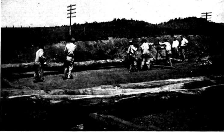
Fig. 13—Handling Poles by Man Power
