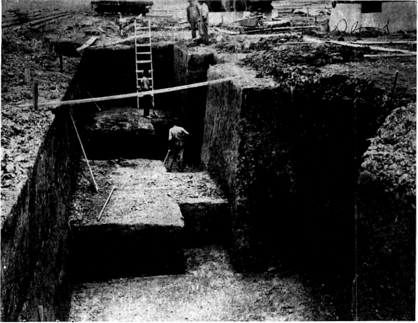
Fig. 24—Excavation for Treating Tanks
