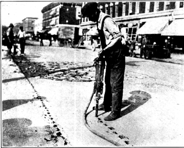
Fig. 22—Air Gun Cutting Asphalt
