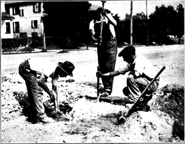
Fig. 23—Manual Method of Breaking Concrete. Contrast with Fig. 21
