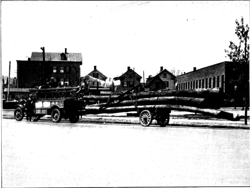
Fig. 11—Balanced Load of Chestnut Poles on Trailer
