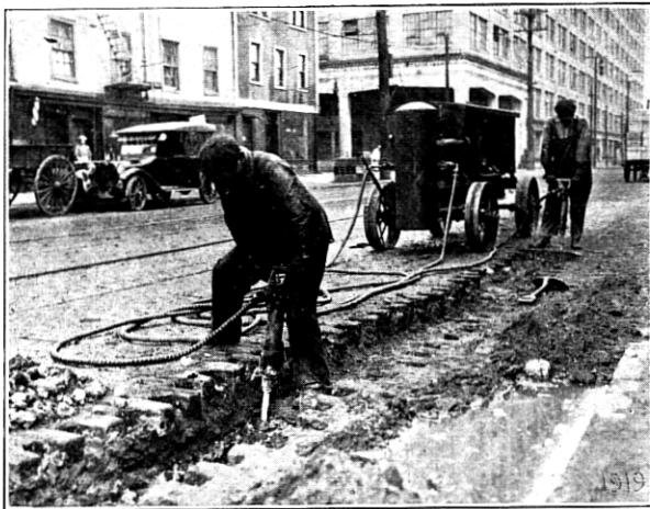
Fig. 21—Removing Granite Blocks and Breaking Concrete Base
