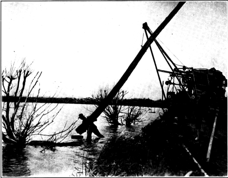
Fig. 5—Derrick Operating Under Difficult Conditions
