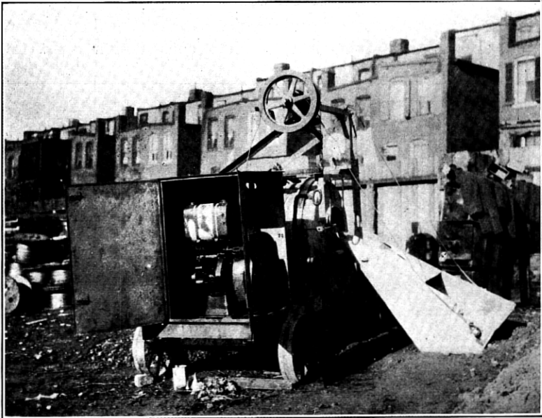
Fig. 13—Concrete Mixer Adapted to Meet Telephone Construction Requirement
