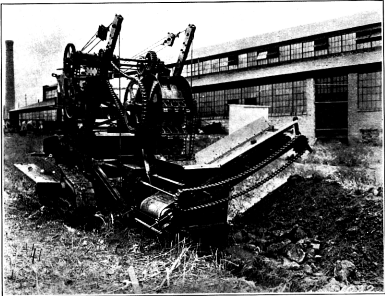
Fig. 16—Light Weight Trenching Machine.
