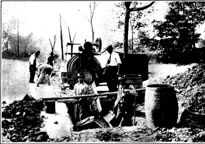
Fig. 14—Pouring Concrete Manhole. Note 4-way Chute for Distribution
