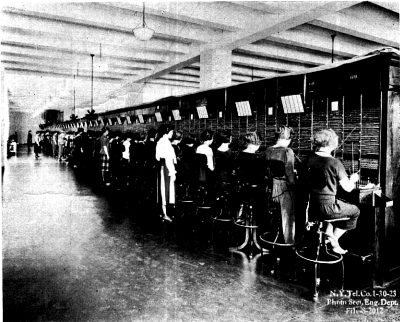
Fig. 2—Modern Type Common Battery Switchboard
