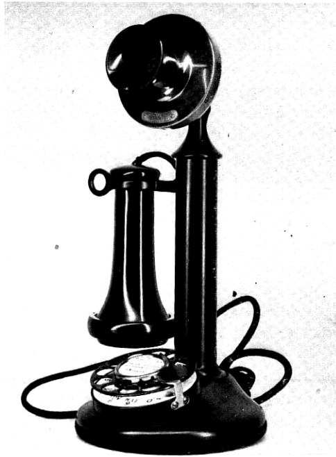
Fig. 5—Desk Stand Equipped with Dial
