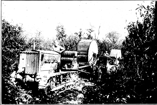
Fig. 12—Tractors Placing Cable Reels in Rough Country
