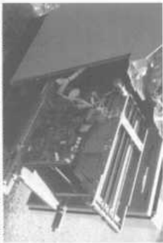
Fig. 3: Lock case w/ change key, alarm wiring & boltwork
